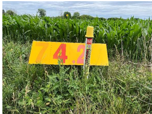
View of Petroleum Pipeline Identifier
